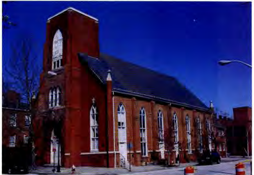
Bell Tower Commons in Baltimore's Otterbein/Sharp-Leadenhall neighborhood involved the adaptive use of a 100-year-old church, resulting in townhouse condominiums. Completed in 1989, Bacon's firm was codeveloper of the project.
